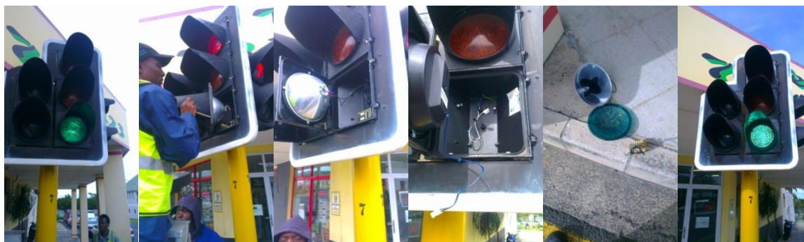
Figure – Upgrade of traffic signal heads to LED
