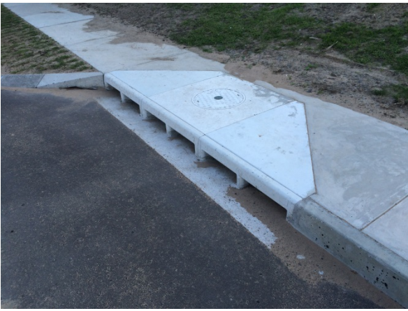
Above: New Polymer Kerb Inlet
