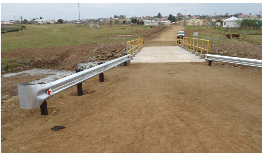
Figure – Ndevana Stream Crossing
